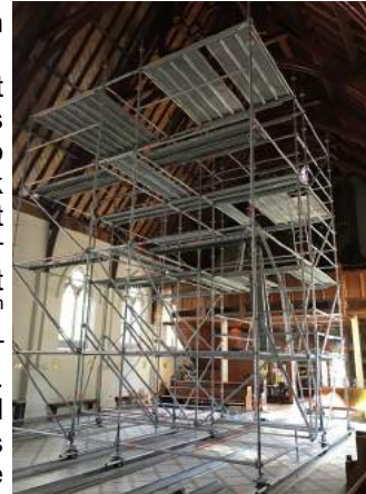
Scaffolding being erected in the church
